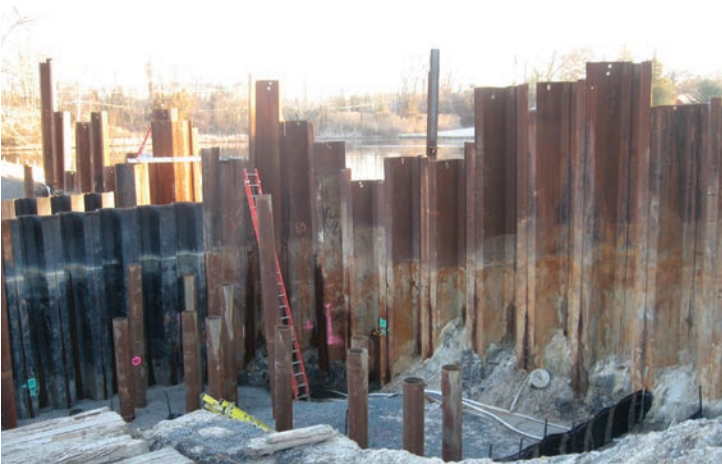
The poles are pounded into the ground, are trimmed and filled with concrete. The piles support the footing that supports the precast arches.
