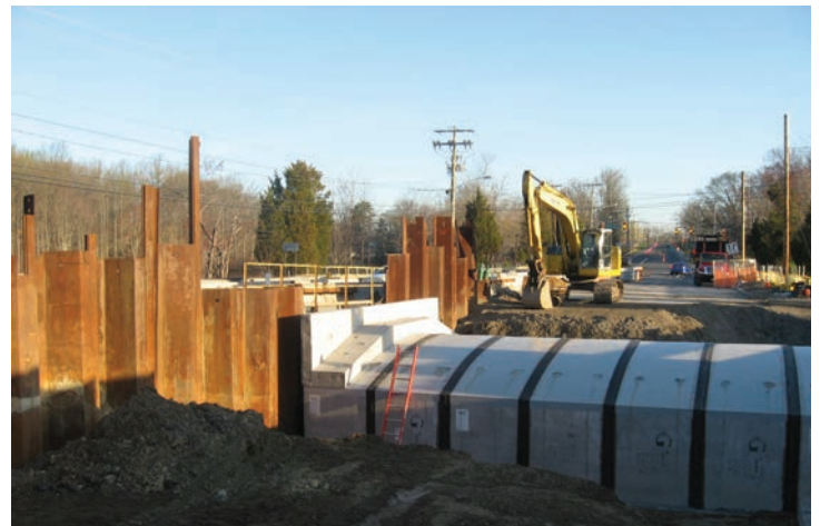
After the bridge arch joints are sealed, the area is backfilled with gravel and specific soils. The final driving surface is created with approximately 10 inches of three different asphalt mixes.
