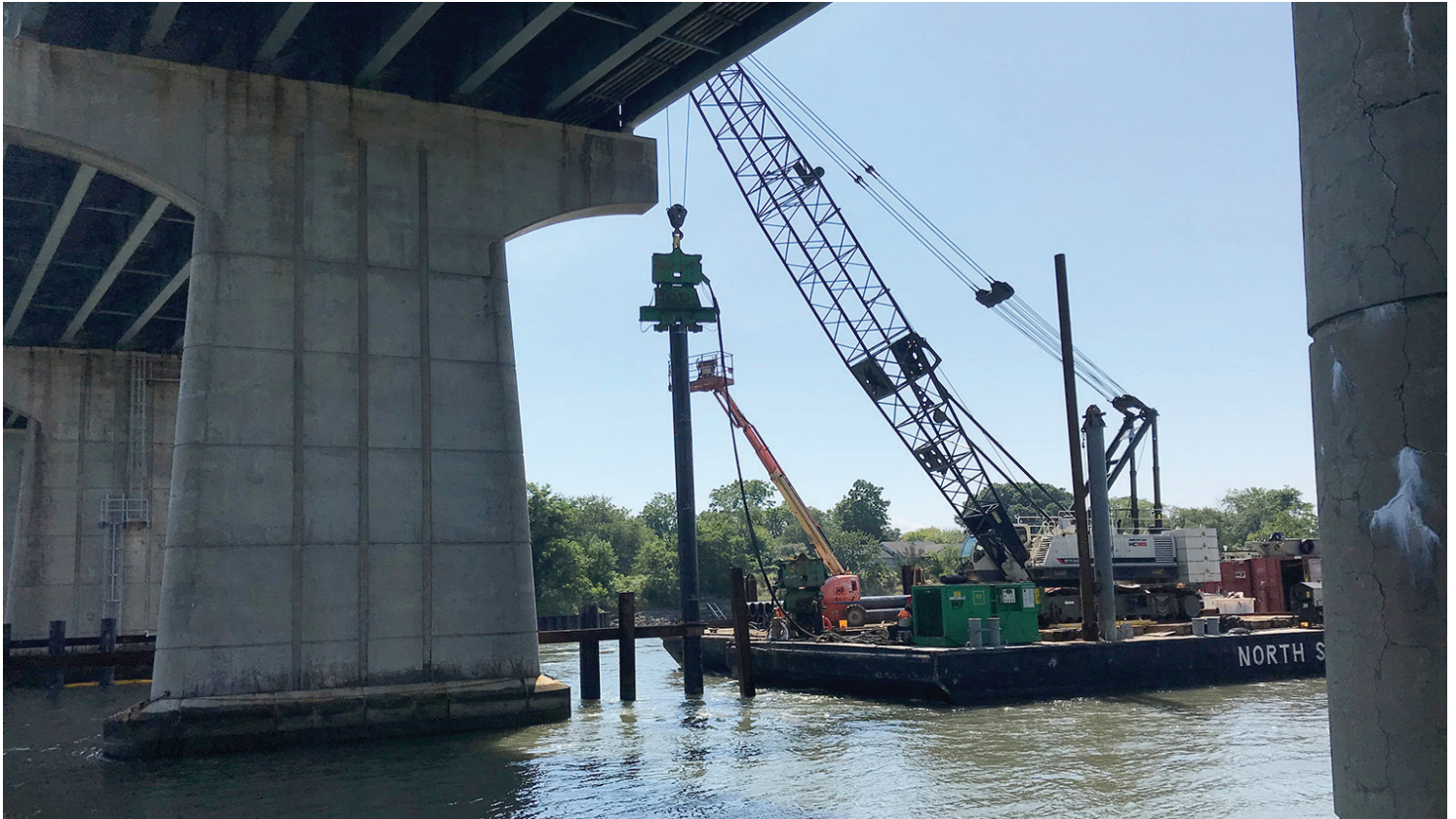
The five-span, 485 foot-long, Route 162 over Cape May Canal structure, received a new fender system built from environmentally friendly, corrosion resistant material.
