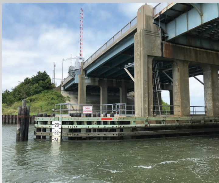
Retroreflective panel on Route 47 over Grassy Sound provides delineation of navigable channel in all weather conditions
