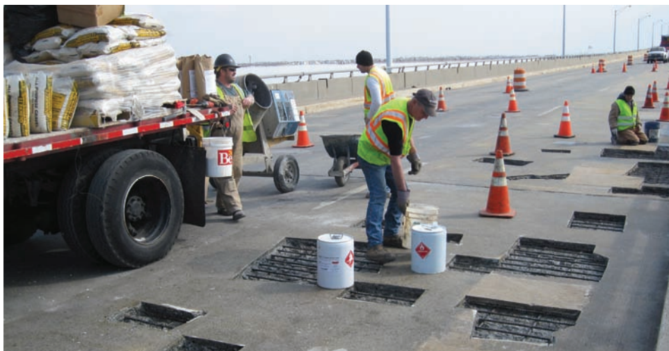
Workers prime all open areas prior to pouring polymer concrete for repairs on Route 37 over Barnegat Bay. Others prepare mixture for polymer concrete.
